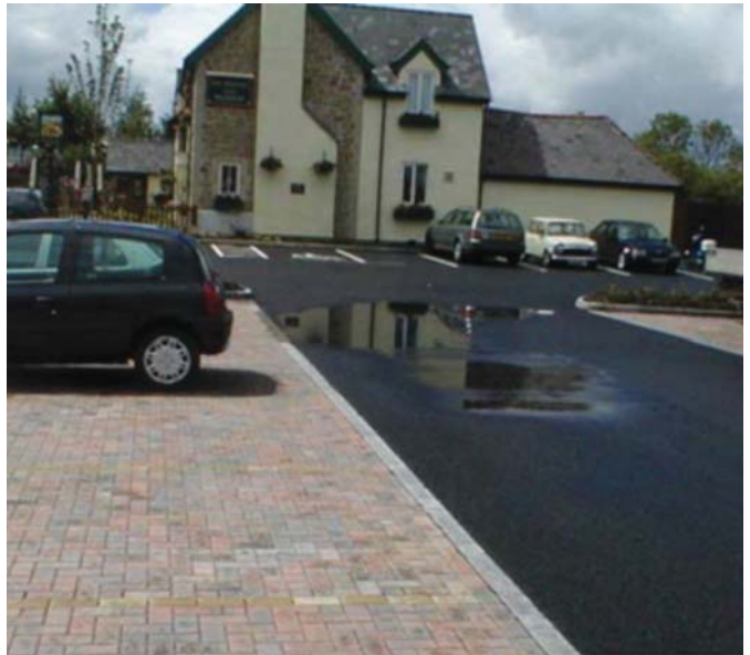
CBPP avoids ponding, unlike conventional sealed paving (above). Rainwater passes straight off CBPP through permeable joints between blocks (below).
