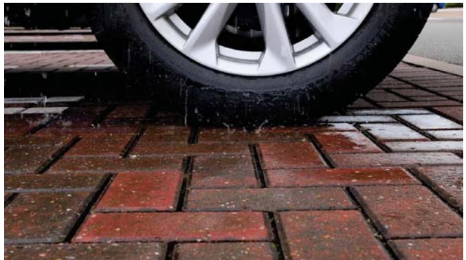
CBPP avoids ponding, unlike conventional sealed paving (above). Rainwater passes straight off CBPP through permeable joints between blocks (below).
