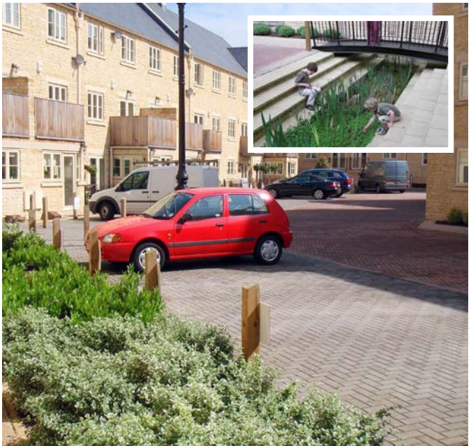
CBPP at this housing scheme in Stamford supplies clean water to landscape features.
