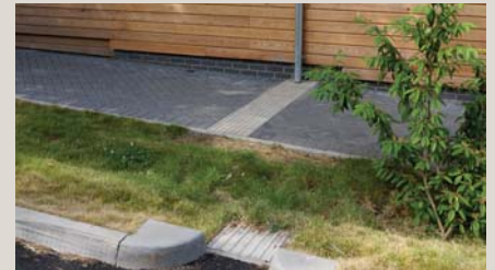
St George's School, Kidderminster - in addition to permeable paving, concrete flags, kerbs and edging have been used for carefully detailed SuDS conveyance, dispersing water and maintaining low flows, such as standard 'bull-nose' concrete kerbs allowing runoff to trickle onto grassed swales.
