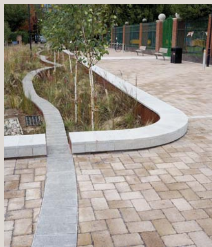
Australia Road, London – concrete block permeable paving laid over an existing road base collects rainwater and gradually discharges it horizontally into planted basins.
