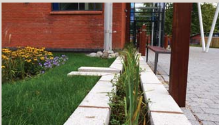
Bewdley School, Worcestershire – standard precast concrete units form rills handling rainwater from conventional concrete block paving and roofs – some via animated water features.
