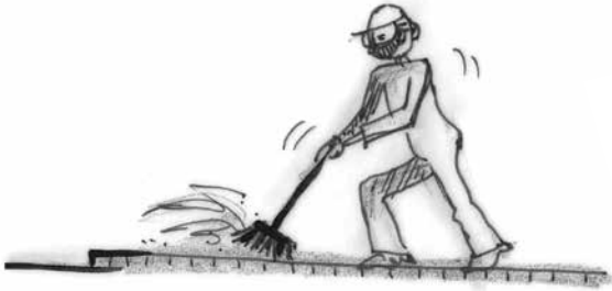
Sweep all debris from pavers before compaction
