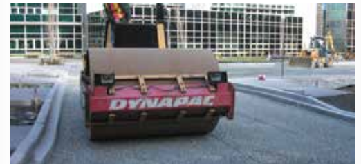
Aggregate base and subbase are spread and compacted; pavers are delivered ready to install. After placement, joints and/or openings are filled with small aggregate. Then pavers are compacted.
