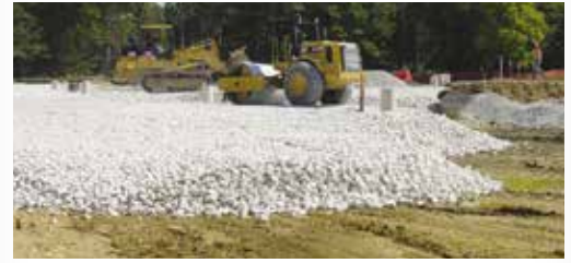
Base construction uses locally available materials.
