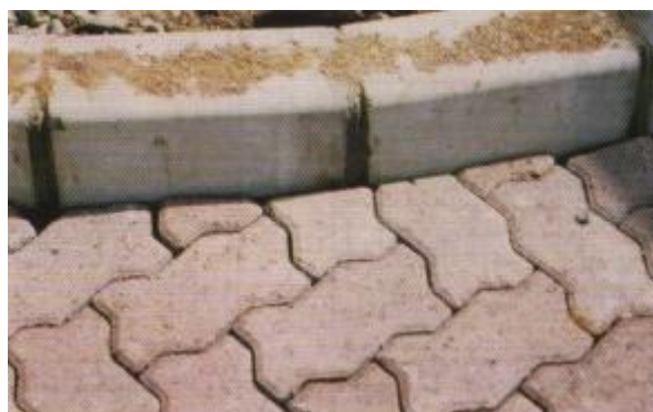
Cutting blocks at edge restraints
