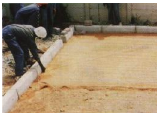
Edge restraints installed before laying commences
